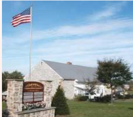
SEESI Office—Lebanon, PA
