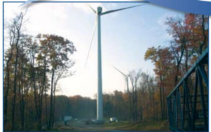
**The turbine blades measure in excess of 150 feet from tip to tip. The towers stand 290 feet high in columns that are more than 12 feet in diameter to accommodate the necessary wind generation and storage equipment.**
